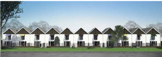
TOP: Artist's impression, terraced units as viewed from the street. BOTTOM: As viewed from the park.
