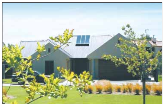
10. Skylight, vents on gables
