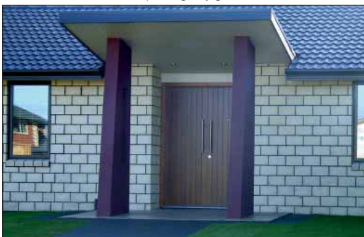
9. Entrance features/columns, double entry doors
