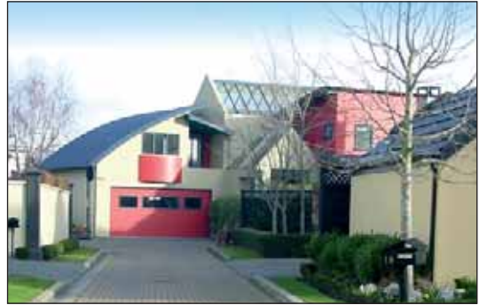
2. Roof line, balcony and skylights
