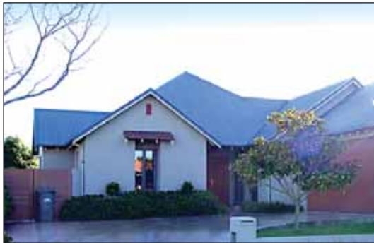
5. Cedar shingles over windows, recessed windows
