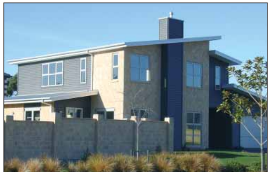
8. Mixed cladding, alternative roofline, feature chimney
